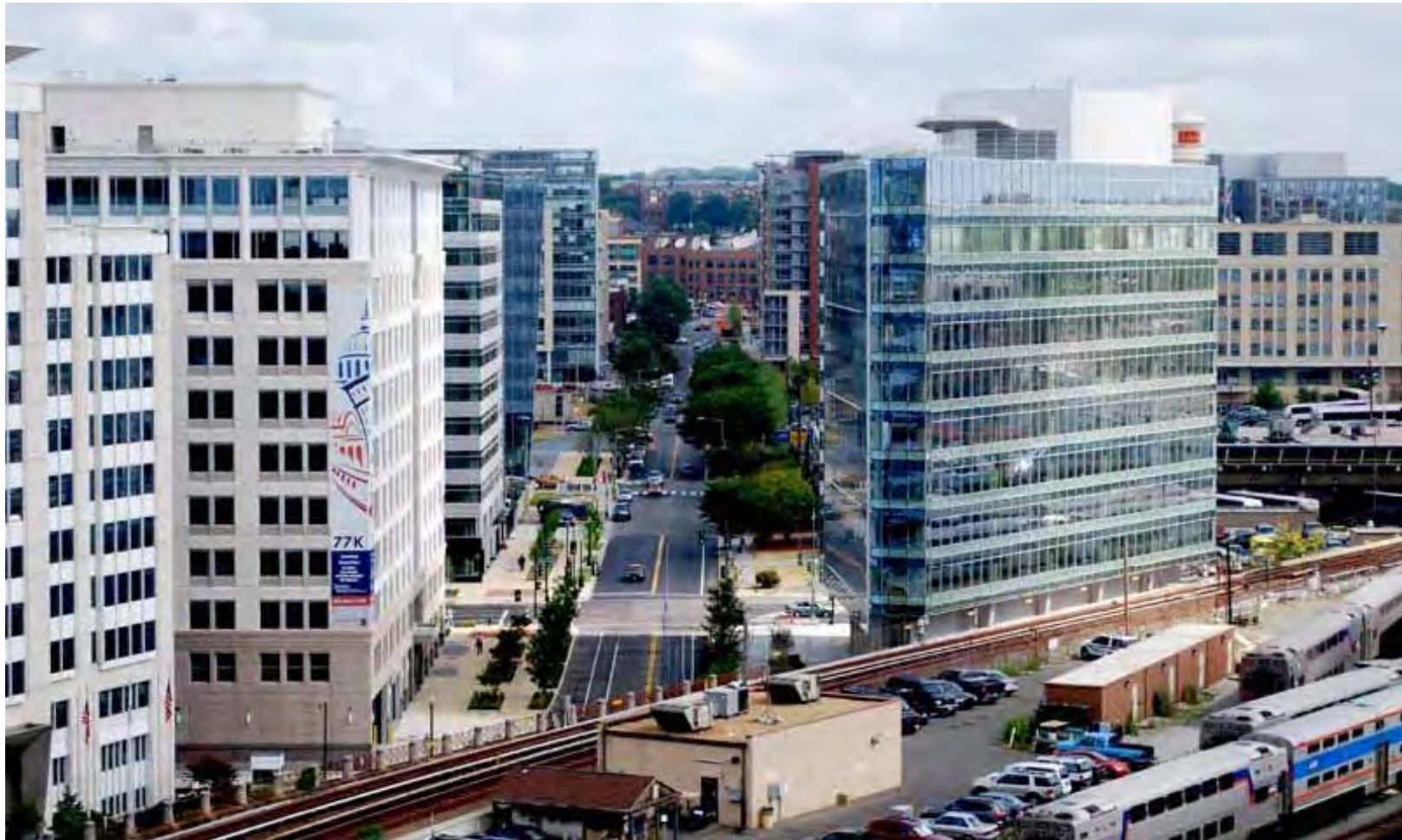
The view up First Street, NE in 2011 shows completed Class A office buildings
